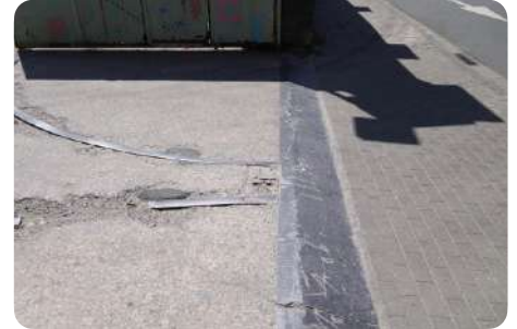
Lowered kerb profile
