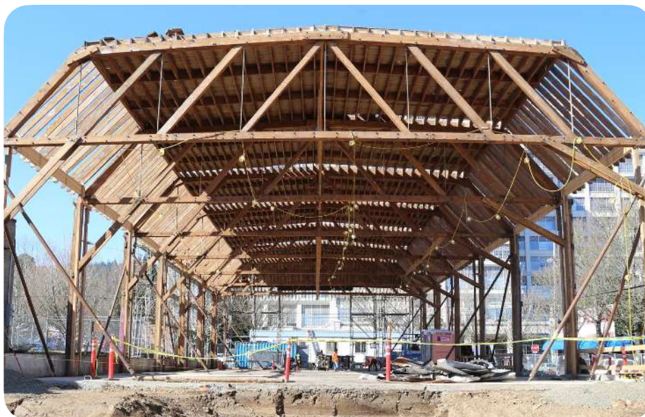
Reuse of 2000 linear meters of solid timber structural elements. Redfox Commons (2019) (USA) © LEVER Architecture
