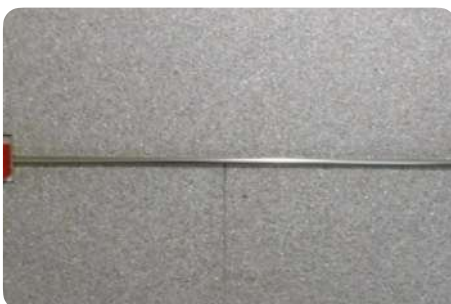
Hollow joint filled with metal elements
