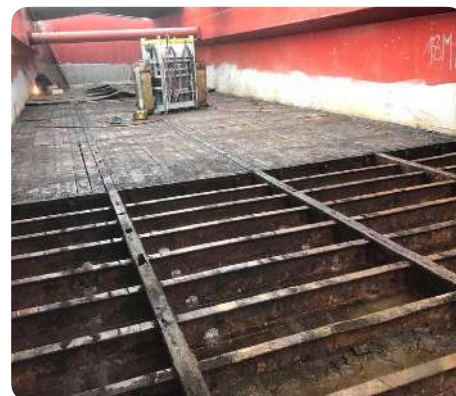
Dismantling of barge holds © historischhout.nl
