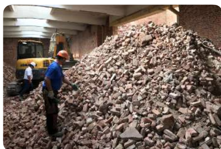
Demolition and reclamation on site. Renovation of the Tour A Plomb, Brussels. © BVDA - Bernard Van Damme Architecte
