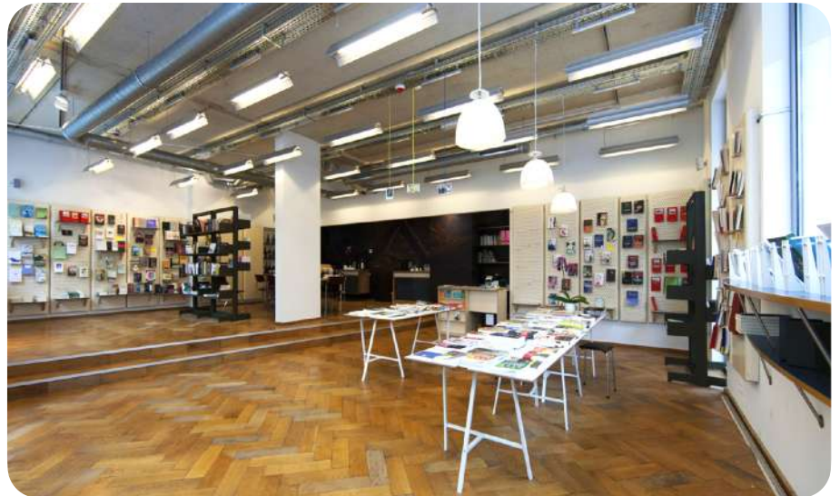
Reclamation of 80 m 2 of oak floorboards, herringbone pattern, Librebook bookstore, Brussels (BE) © Rotor
