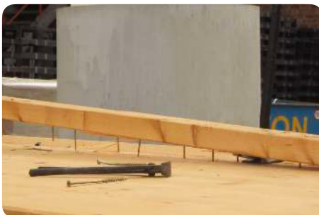
Removal of metal parts
