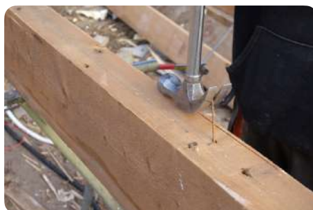
Removing metal parts
