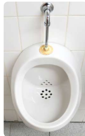
Suspended urinal with siphon-action, with rim, visible top feed and integrated waste.
