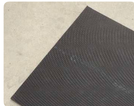
Back of a carpet tile laid without glue.
