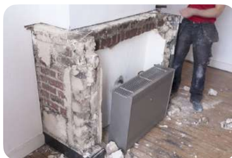
Dismantling the mantelpiece
