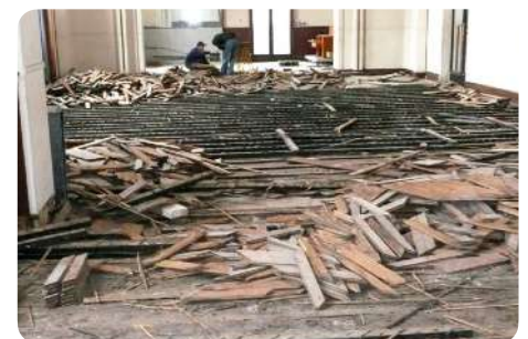
Removal of a wooden floor nailed to joists
