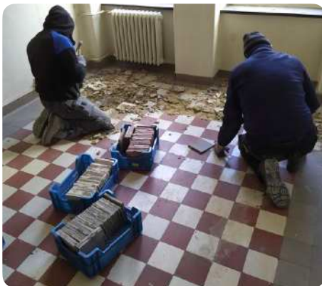
Careful dismantling of tile floor
