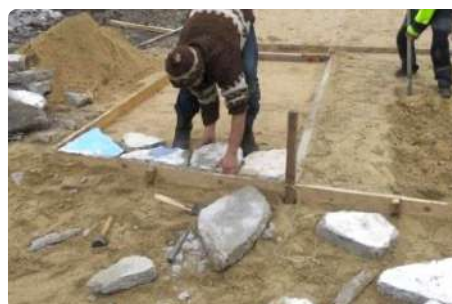
The "Opus uncertum" of Clos Saint Lazare in Stains (FR), 2017. The concrete resulting from the demolition of a residential building built in 1959 was reused on site to cover the ground of the outdoor spaces.
