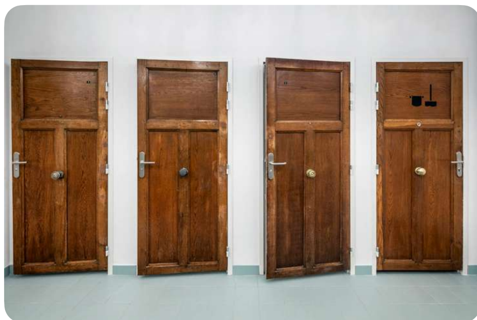
Reuse of panelled wooden doors © Cyrus Cornut, Grande Halle de Colombelles, WIP. Architects: Encore Heureux (FR)
