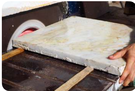
Removal of mortar residues from the edge using a lapidary machine
