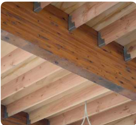
Reused glue lam beams
