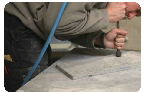
Bush hammering of slabs
