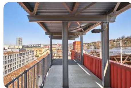
Installation of beams
