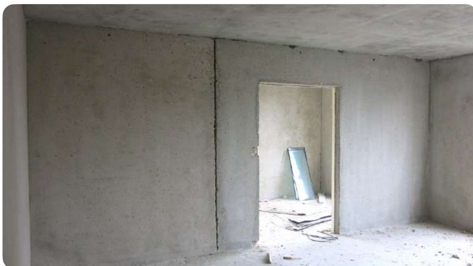
Prefabricated walls after stripping of interior linings and removal of asbestos from surfaces, before demolition or deconstruction of the building.
