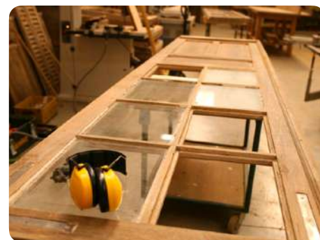
Replacement of glazing elements
