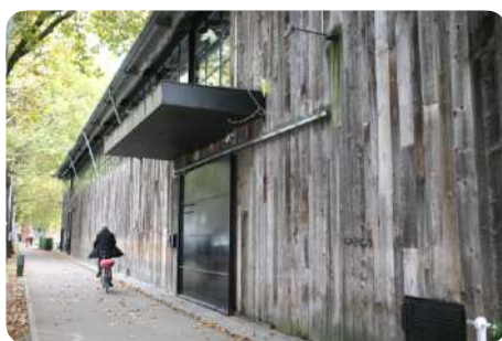
Re-use of 800 m 2 of barnwood for exterior cladding and interior panelling. Quay01 (K-nal), Brussels (BE) © Jean-Paul Hermant architectes https://opalis.eu/fr/projets/bardage-quay01-k-nal
