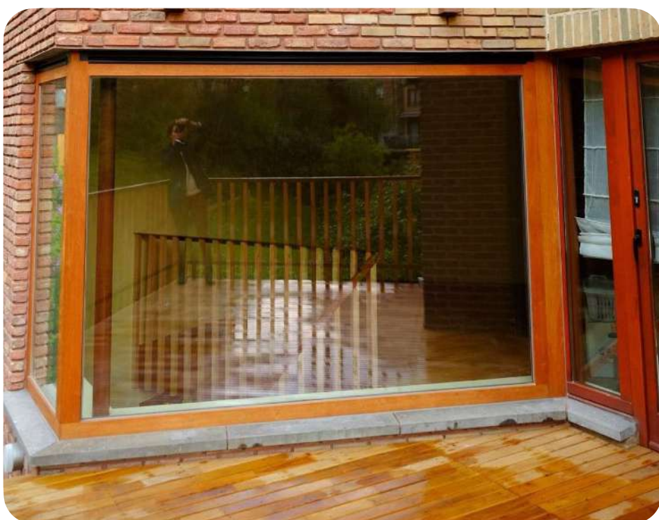
Reusing old coping stones for window sills © Sophie Boone
