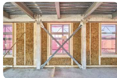
Installation of beams
