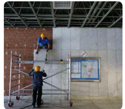
Careful dismantling of marble wall panels
