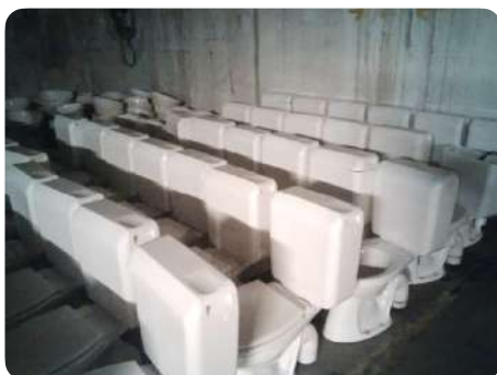
Removal of toilet bowls for reclamation
