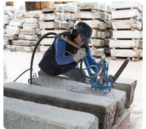
Kerb finishing by bush hammering © Carrière de Bonneuil-sur-Marne
