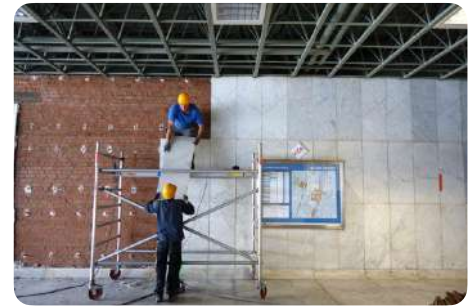
Removal of marble slabs
