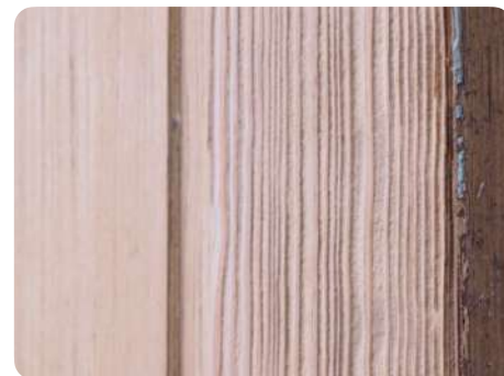
The sanding of the wooden elements widens the grooves in wood
