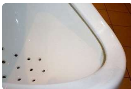
Traces of scale on the rim, after cleaning
