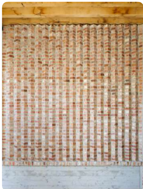
Interior wall facing in reclaimed bricks. Zonnige kempen. (BE)
