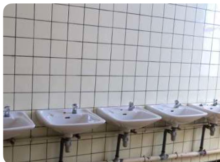
Wall tiles and sinks before dismantling
