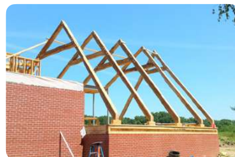
Reclamation of structural beams © yr-architecture (USA)
