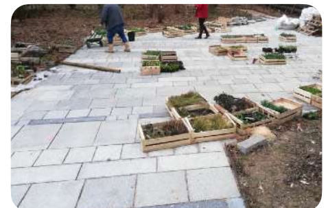
Reuse of granite and Hainaut stone slabs of various sizes and shapes, recovered from the City of Paris warehouse. Square de la biodiversité, Paris (FR) © Perrine Henault, Atelier NOUS
