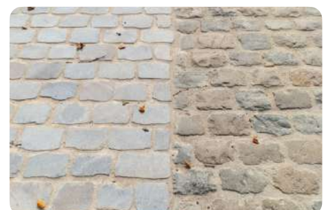
Installation of sawn / rough pavers
