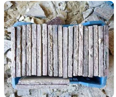
Few mortar remains after removal (hybrid mortar)
