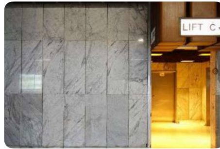
Marble slab wall covering
