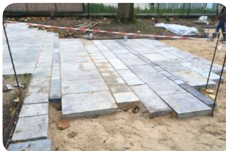
Reuse of granite and Hainaut stone slabs of various sizes and shapes, recovered from the City of Paris warehouse. Square de la biodiversité, Paris (FR) © Perrine Henault, Atelier NOUS
