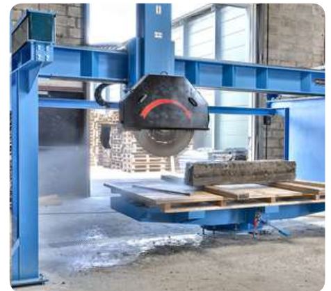
Kerb sawing © Carrière de Bonneuil-sur-Marne
