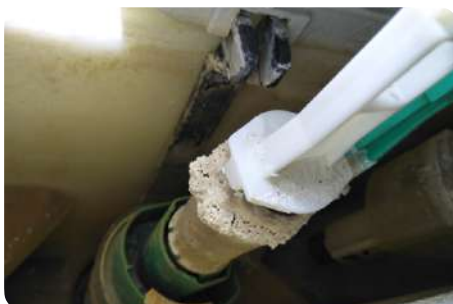
Scaling of the flushing mechanism
