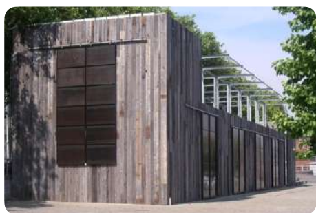
Re-use of 800 m 2 of barnwood for exterior cladding and interior panelling. Quay01 (K-nal), Brussels (BE) © Jean-Paul Hermant architectes https://opalis.eu/fr/projets/bardage-quay01-k-nal
