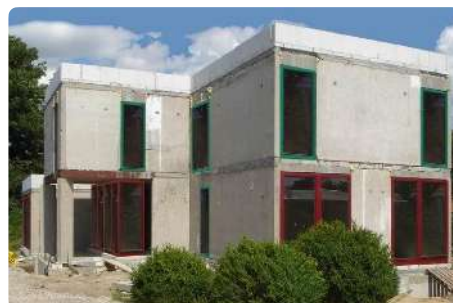
The "plattenbau houses" Das Recyclete Haus. Built in the early 2000s in Mehrow (Berlin), these houses were constructed from prefabricated concrete slabs from the deconstruction of apartment blocks in East Berlin ("plattenbau"). The prefabricated slabs were removed and reused as floor slabs and load-bearing walls. © Bureau d'architecture Concluz.
