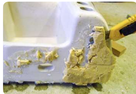
Removal of adhesive remains
