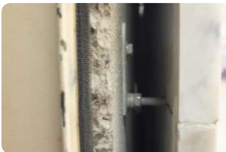
Fastened stone cladding
