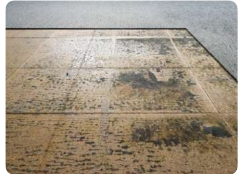
Residual glue on the upper face of the coverings.
