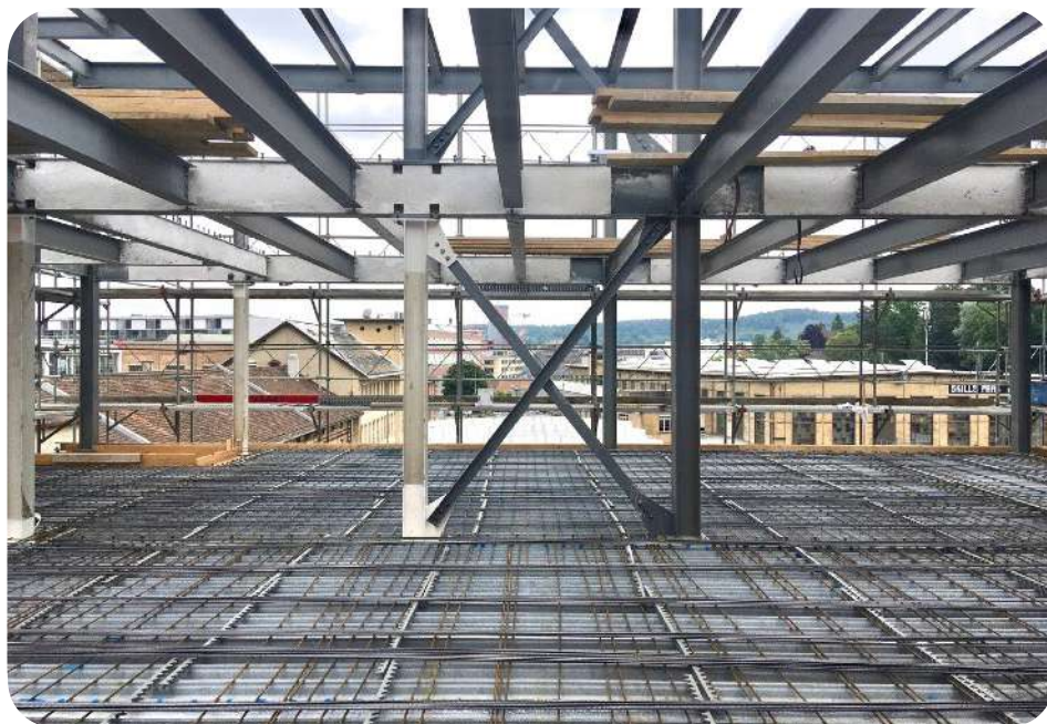
Installation of beams
