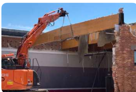
Removal of glulam beams
