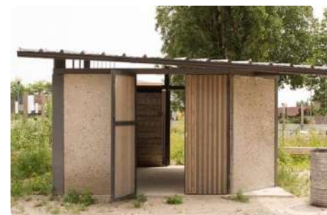
The pavilion of the Fabrique du Clos in Stains. During the demolition of a housing complex in Stains, some of the concrete elements were reclaimed on the site. The extracted concrete walls were sawn on site and reused as non-load-bearing walls for a bicycle room. The paving of the floors of the outdoor areas was also made from raw concrete blocks. Contracting authority: Seine-Saint-Denis Habitat. Design: Bellastock. Stains (France), 2017 © Alexis Leclercq
