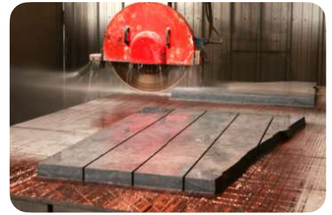
Cutting stone elements
