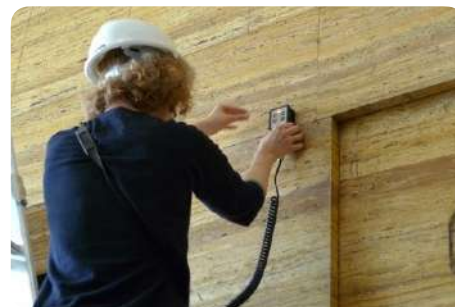
Searching for metallic anchoring elements of a natural stone facing using a pachometer. © CSTC
