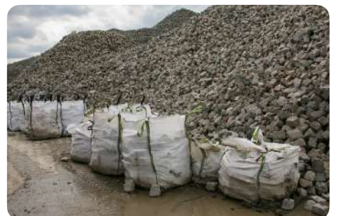
Storage of paving stones in big bags
