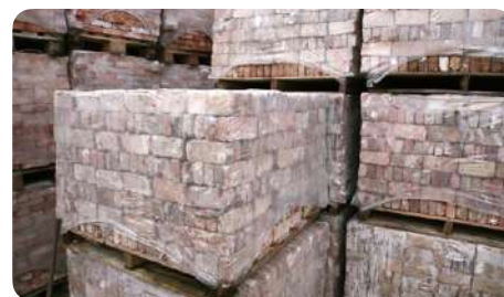
Storage of sorted and cleaned bricks on covered pallets
