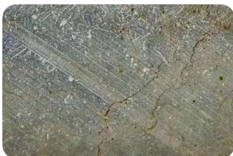
Superficial cracking
