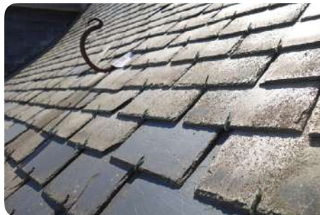
“Original” slates and “repair” slates.
