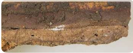
Mortar remains on edges and back side
