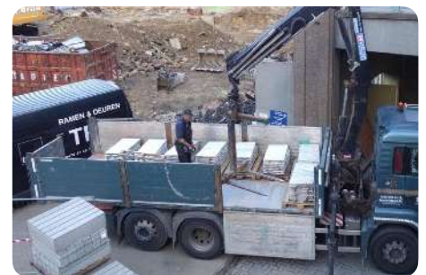
Loading and transporting slabs
