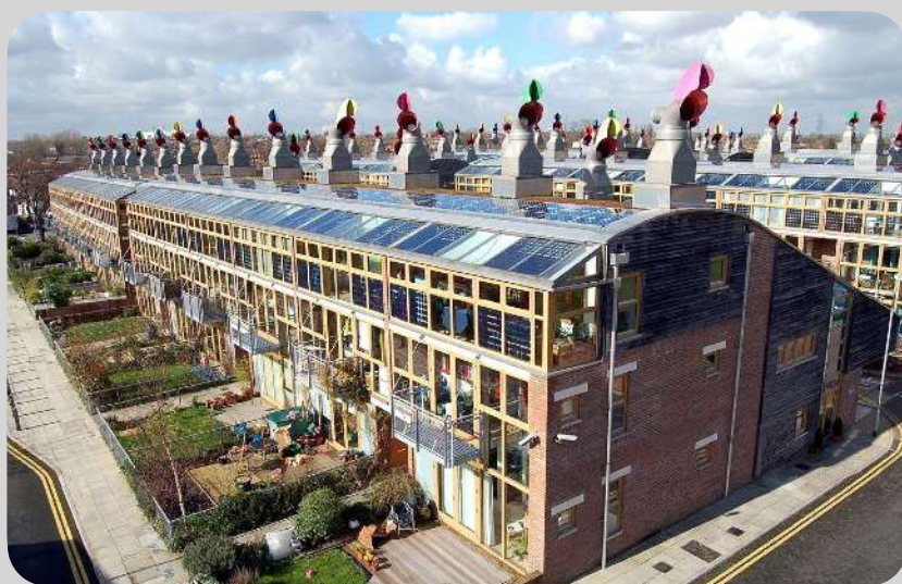
Bedzed Project (2002), Hackbridge (UK). Reuse of 95 tonnes of steel © Bill Dunster Architects, ZedFactory
