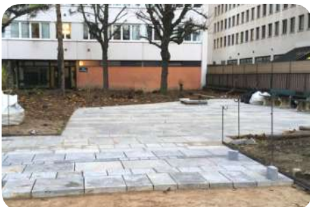
Reuse of granite and Hainaut stone slabs of various sizes and shapes, recovered from the City of Paris warehouse. Square de la biodiversité, Paris (FR) © Perrine Henault, Atelier NOUS
