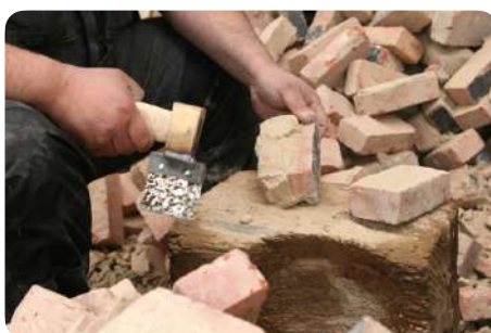
Manual cleaning of mortar remains
