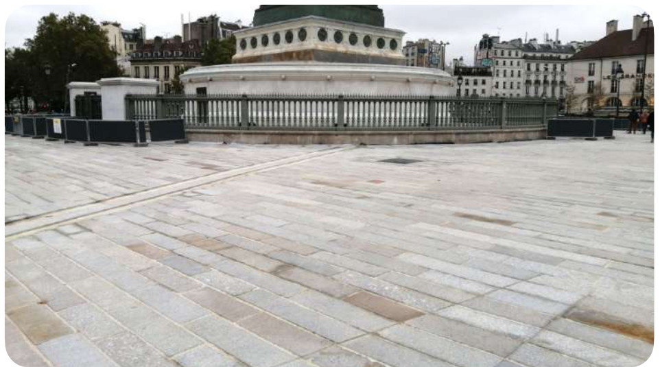
Place de la Bastille, Paris. Reclamation of 10,000 old kerb stones sawn in half to be transformed into flagstones (FR). © Benjamin Randow
