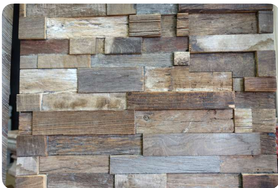
Multi-species interior panelling with boards of variable dimensions.
