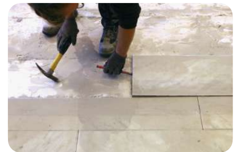
Removing the slabs
