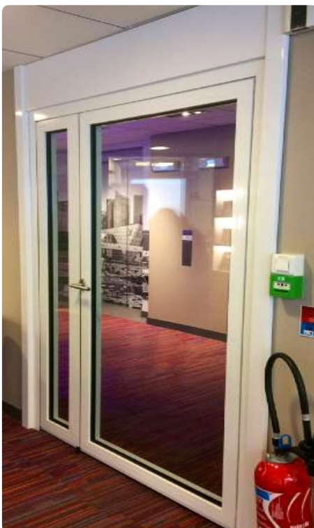
Example 2. Before reclamation
