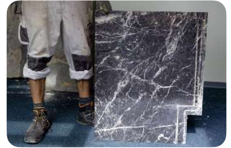
Sealant and cutting for housing the shelf © Frédéric Uyttenhove
