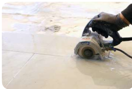
Sawing joints
