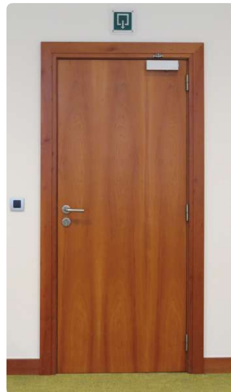
Example of a fire door
