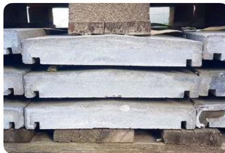
Double inclined surface coping © Rotor DC
