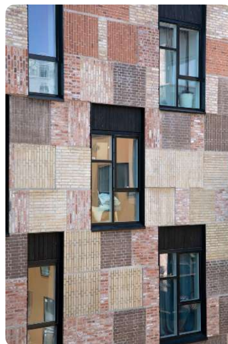
Reuse of brick modules. The Resource Rows. © Lendager Group (DK)
