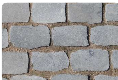
Installation of sawn setts
