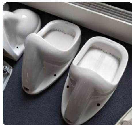
Removal of urinals
