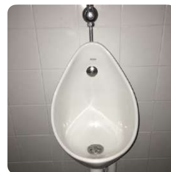
Suspended flushing urinal, diffuser and metal plug, visible supply and outlet. © backacia.com
