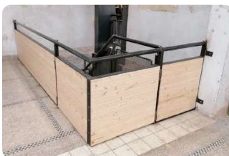
Conversion into guard railing, Brussels (BE) © Zinneke
