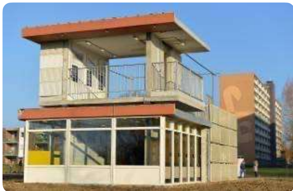
Super Local Project. This experimental project carried out in 2017 in the Netherlands implemented a reclaim process of three-dimensional concrete modules extracted from an old housing building, for the construction of individual houses. The modules consist of slabs and walls, which were sawn before being crane-mounted and transported by truck to the nearby reclaim site. Client: HEEMWonen. Architect: SeC Architects. Contractor: Jongen Construction. Research unit: Zuyd University of Applied Sciences, Research group SURD.
