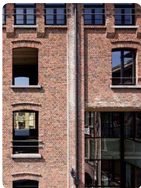
On-site reuse of bluestone sills, reconversion of the former Belle-Vue breweries, Brussels, (BE) © François Lichtlé, L'Escaut Architectures. https://opalis.eu/fr/projets/reconversion-des-anciennes-brasseries-belle-vue
