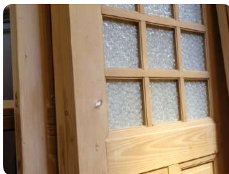
Panel door stripped and sanded
