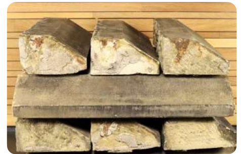
Sloped surface coping © Willmow Reclamation & salvage
