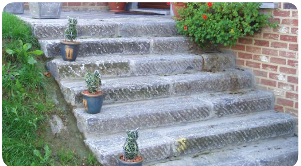
Reclamation of kerb stones for staircase steps (FR). © Noblema
