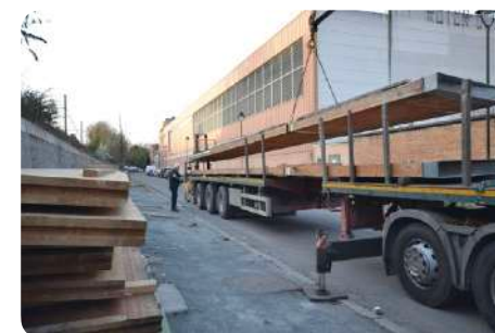
Transport of glulam beams
