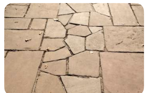
Mix of square York sandstone slabs and "broken" slabs laid in Opus Incertum, Holland Park, London (UK) © Thornton Kay/Salvo
