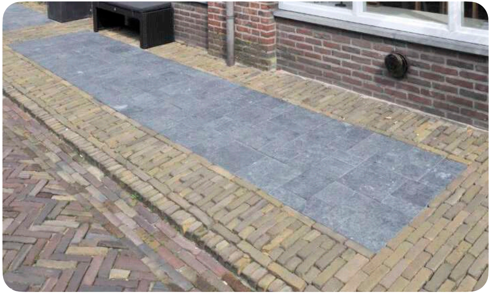
Renovation of pavement with reclaimed clay pavers, Bergen (NL), 2020 © Stone Base
