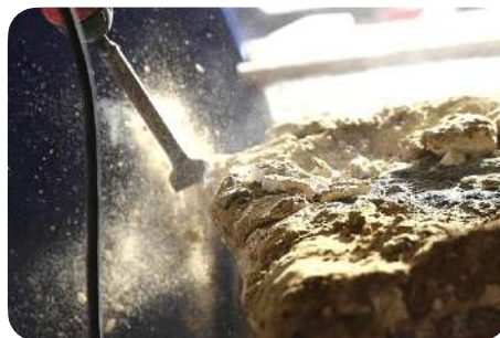
Removal of mortar residues with a pneumatic chisel © De Opkamer
