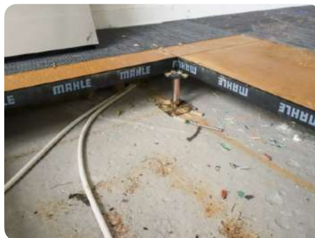
Self-supporting raised floor. Agglomerated wood-based coverings, with a textile covering (carpet tiles).
