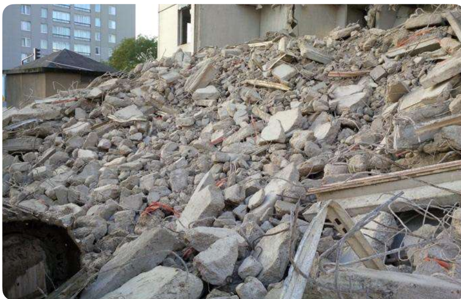
Concrete rubble deposit from the demolition of a tower at Clos Saint Lazare in Stains (FR).
