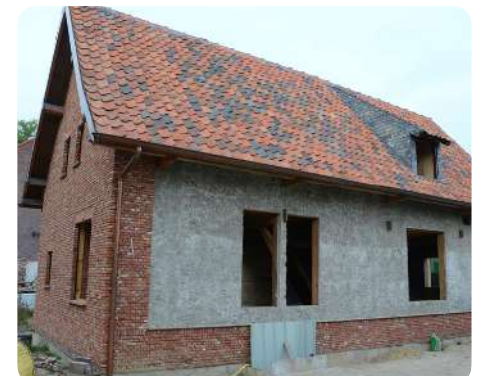
Example of reused clay roof tiles (BE) © deoudedakpan.be
