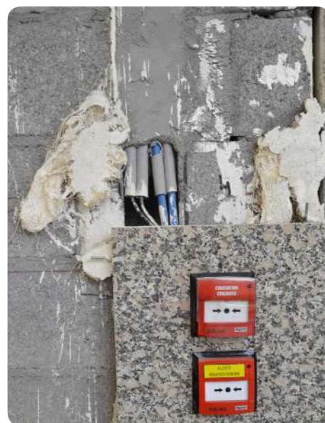
Removal of interior facing slabs in granite
