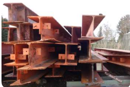
Recovered beams with welded connections © Gebruikte bouwmaterialen Weert
