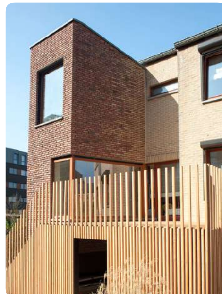
Extension of a single-family house. Reclaimed brick façade cladding. Brussels (BE) © Sophie Boone for VLA-Architecture
