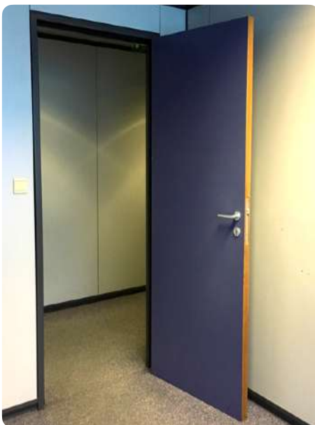
Example 1. Before reclamation
