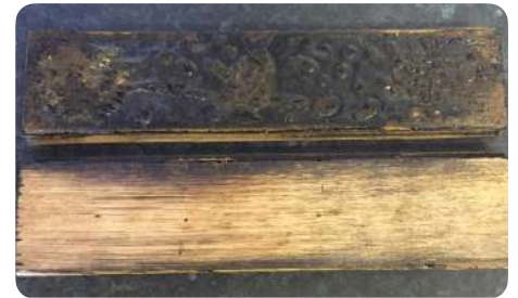
Cleaning of bituminous adhesive residues © www.parquetbitumenremoval.co.uk
