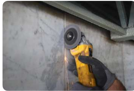
Cutting fasteners
