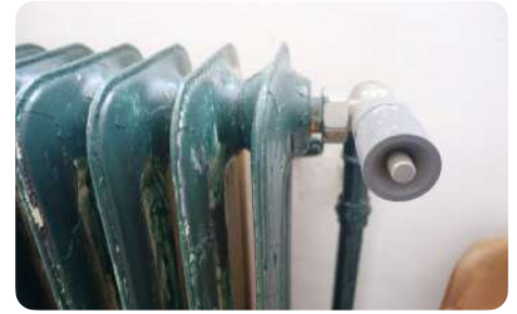
Certain sheet steel radiator models can be confused with cast iron radiators.
