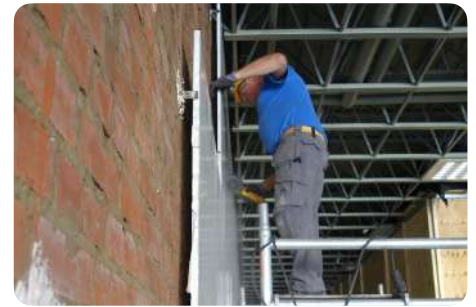
Fixing by hooks
