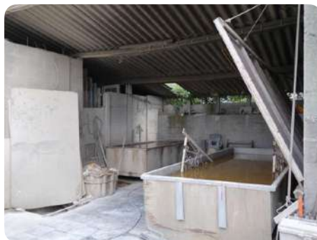
Chemical soaking plant
