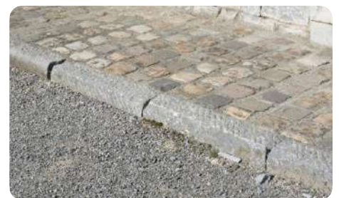
Blue stone “town” kerbs. Road development. © Carrière de la Hazotte
