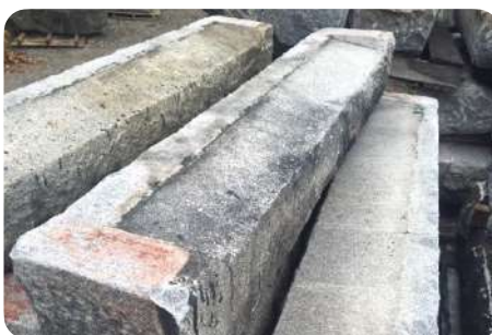
Granite window sill © Stone of New England
