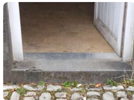
Blue stone door threshold (limestone)
