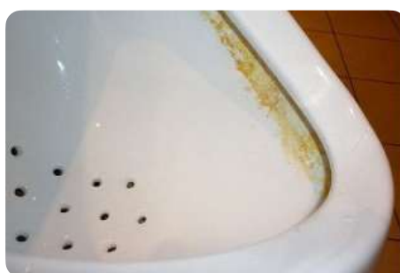
Traces of scale on the rim, before cleaning
