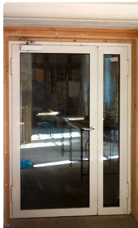
Example 2. After reclamation
