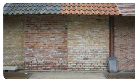
Showroom of a reseller of reclaimed bricks. Enhancement of the different models, with joints of varying nature and thickness
