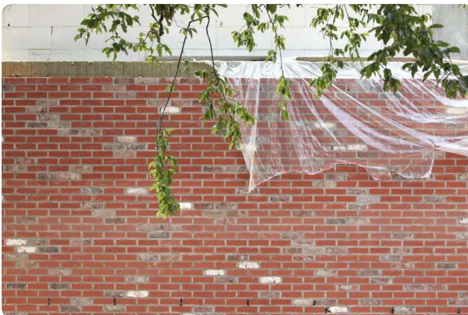
Mixture of reclaimed bricks and new bricks. Folklore Museum, Mouscron (BE). © V+ architectes
