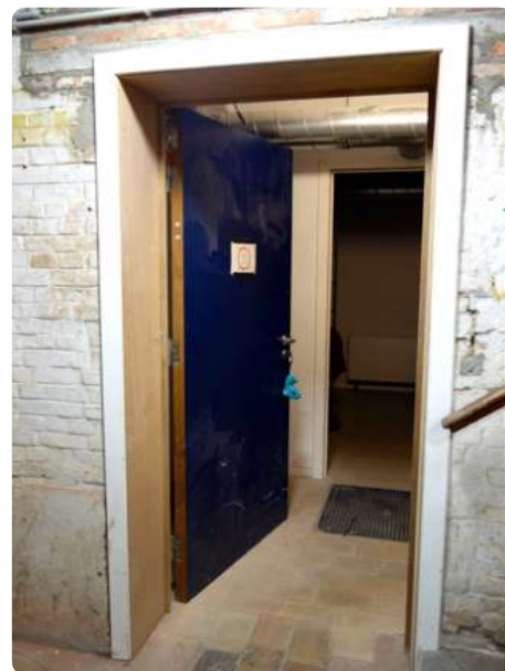
Example 1. After reclamation
