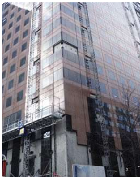
Reclamation of 5300 m 2 of red granite slabs from the façades of the Tour Cèdre in La Défense, Paris (FR). © Incomex http://pierre-reemploi.com/offre/granit-rouge-de-facade-nr01/
