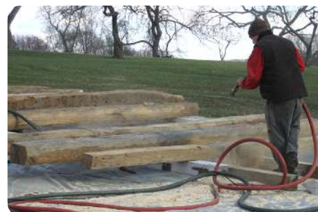
Timber cleaning © yr-architecture
