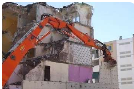
The pavilion of the Fabrique du Clos in Stains. During the demolition of a housing complex in Stains, some of the concrete elements were reclaimed on the site. The extracted concrete walls were sawn on site and reused as non-load-bearing walls for a bicycle room. The paving of the floors of the outdoor areas was also made from raw concrete blocks. Contracting authority: Seine-Saint-Denis Habitat. Design: Bellastock. Stains (France), 2017 © Alexis Leclercq
