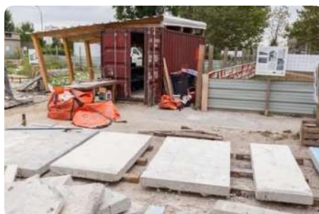
The pavilion of the Fabrique du Clos in Stains. During the demolition of a housing complex in Stains, some of the concrete elements were reclaimed on the site. The extracted concrete walls were sawn on site and reused as non-load-bearing walls for a bicycle room. The paving of the floors of the outdoor areas was also made from raw concrete blocks. Contracting authority: Seine-Saint-Denis Habitat. Design: Bellastock. Stains (France), 2017 © Alexis Leclercq
