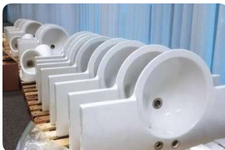
Removal of washbasins for reclamation
