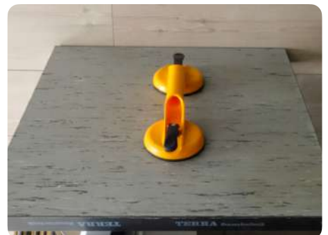
Removal of the coverings using a suction cup
