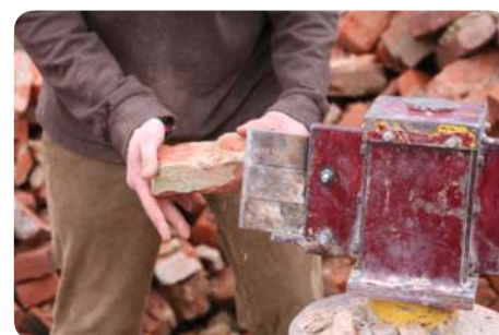
Mechanical cleaning of mortar remains
