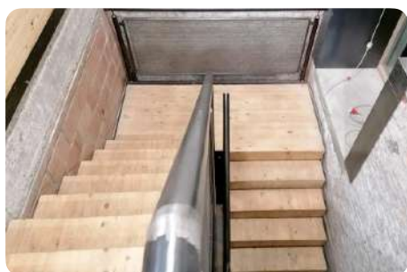
Conversion into stair treads, Brussels (BE) © Zinneke
