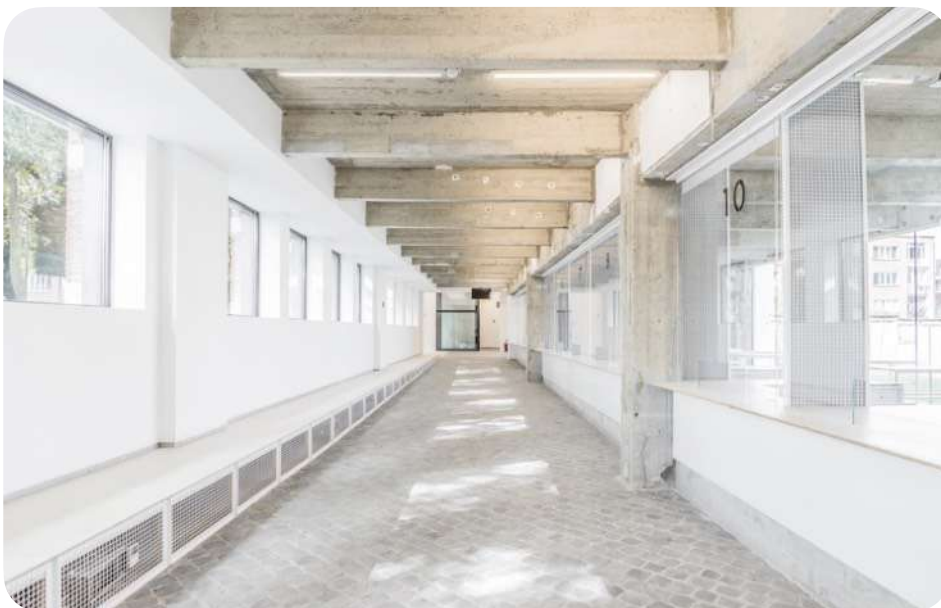
Hergebruikkasseien. Project "Charles Malis" in Molenbeek, Brussel (BE) (Architekten.: Mamout + Willocx + LD2) © Studio Fiftyfifty
