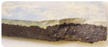
Carreau "ciment" bicouche
