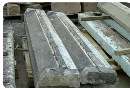
Traces de mortier © valleyreclamation.co.uk
