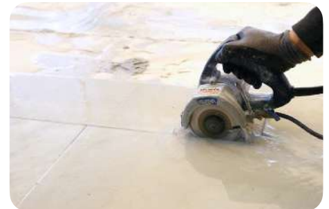
Sciage des joints
