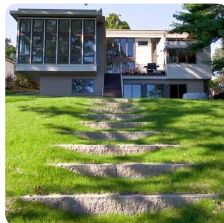
Lower Mystic Lake House (USA). Reclamation of stone kerbs. © matthew-cunningham.com
