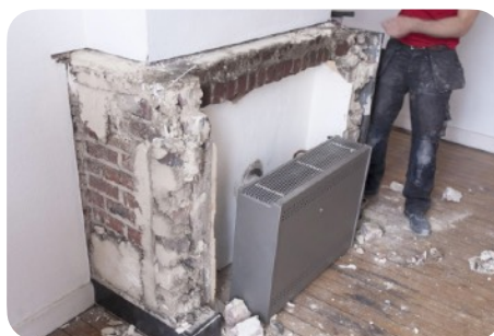
Dismantling the mantelpiece
