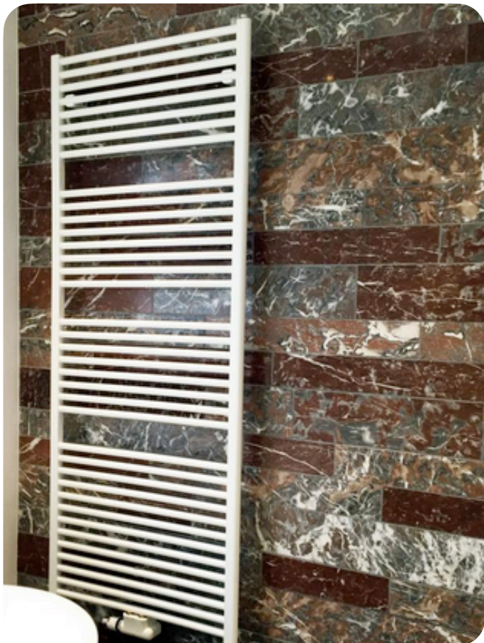
Wall covering from window shelves (BE). © Manugryson architecten
