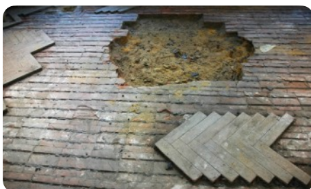
Reclamation of 50 m 2 of broken-batten floorboards. The planks were sawn through to remove the old bitumen glue. They were then reworked in order to be re-installed (glued installation) with a Hungarian herringbone pattern, Boom (BE) © Atelier Passe Partout
