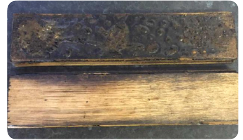
Cleaning of bituminous adhesive residues © www.parquetbitumenremoval.co.uk
