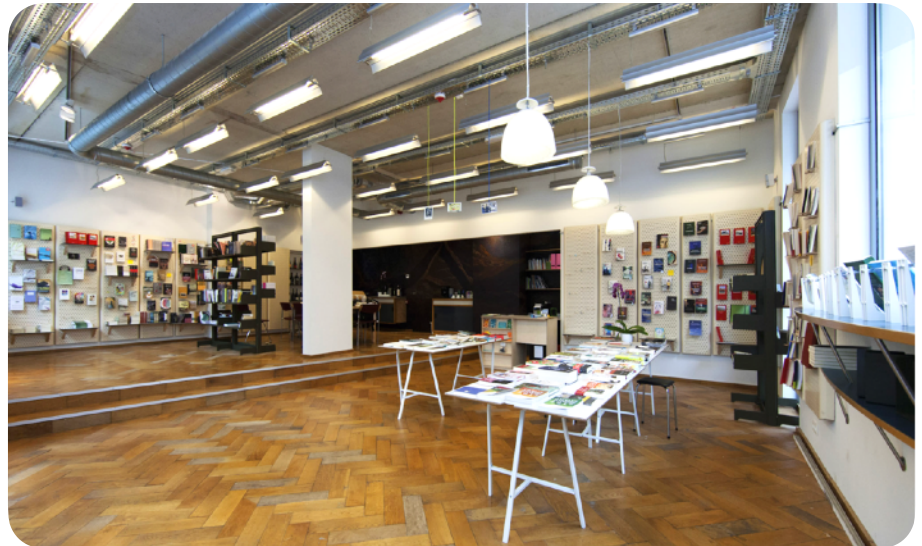
Reclamation of 80 m 2 of oak floorboards, herringbone pattern, Librebook bookstore, Brussels (BE) © Rotor
