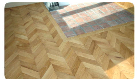
Reclamation of 50 m 2 of broken-batten floorboards. The planks were sawn through to remove the old bitumen glue. They were then reworked in order to be re-installed (glued installation) with a Hungarian herringbone pattern, Boom (BE) © Atelier Passe Partout
