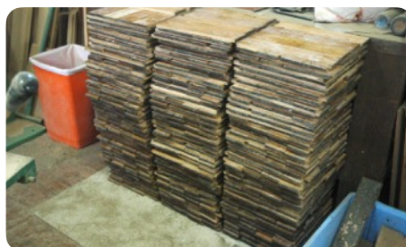
Reclamation of 50 m 2 of broken-batten floorboards. The planks were sawn through to remove the old bitumen glue. They were then reworked in order to be re-installed (glued installation) with a Hungarian herringbone pattern, Boom (BE) © Atelier Passe Partout
