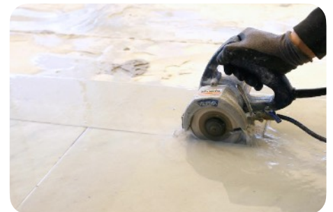
Sciage des joints
