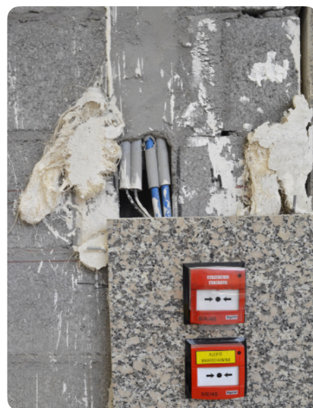
Removal of interior facing slabs in granite
