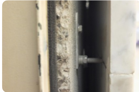
Fastened stone cladding
