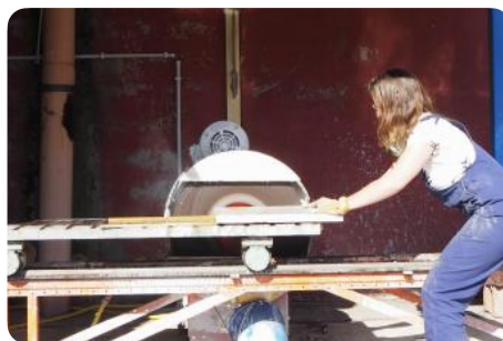
Removal of grout residues from the edge using a lapidary machine
