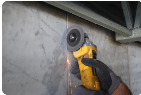
Cutting fasteners
