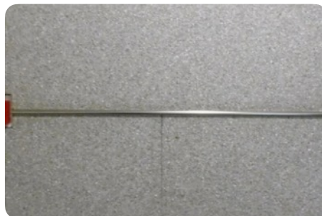
Hollow joint filled with metal elements
