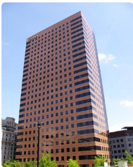
Reclamation of 5300 m 2 of red granite slabs from the façades of the Tour Cèdre in La Défense, Paris (FR). © Incomex http://pierre-reemploi.com/offre/granit-rouge-de-facade-nr01/
