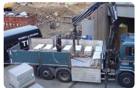
Loading and transporting slabs
