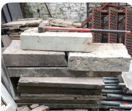
Blue stone exterior coping stones reused for the creation of a terrace, Brussels (BE) © VLA architecture https://www.guidibatimentdurable.brussels/fr/reemploi.html?DC=10994
