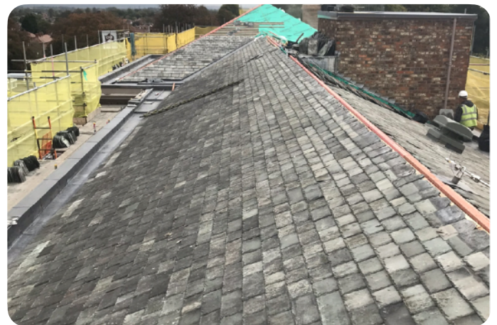
Slate reused and re-installed on the roof © thereclaimedcompany.co.uk
