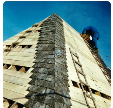
Nailed installation of reclaimed slate, thick model, mixed installation with decreasing gauge (FR) © Sarl Ritouet
