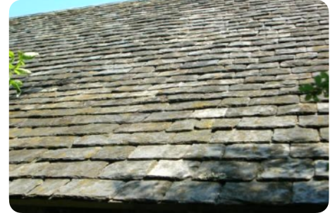
Nailed installation of reclaimed slate, thick model, mixed installation with decreasing gauge (FR) © Sarl Ritouet
