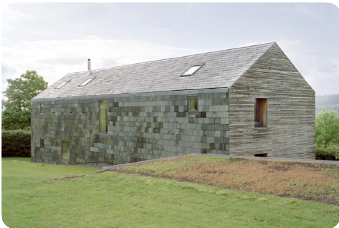
Reclaimed slate roof and cladding, Ty Pren project (UK), Feilden Fowles architects © David Grandorge
