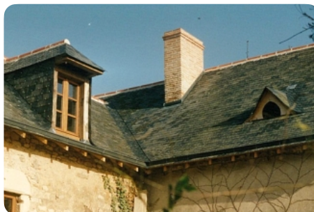
Hook laying of reclaimed slate, fine model (FR) © Sarl Ritouet
