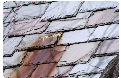
Mineral inclusions and traces of rust. © nachi.org
