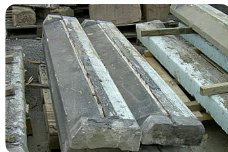
Traces de mortier © valleyreclamation.co.uk
