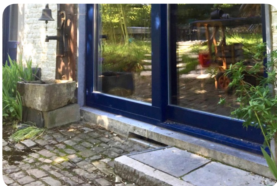
Reuse Inspiration. Sliding sash sill consisting of two old window sills cut to the right size and cut to provide ventilation of the cellar (hole in the centre) © Sophie Boone
