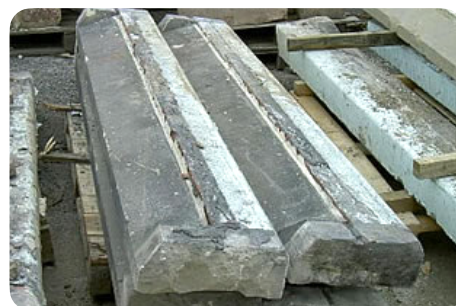
Traces of remaining mortar © valleyreclamation.co.uk
