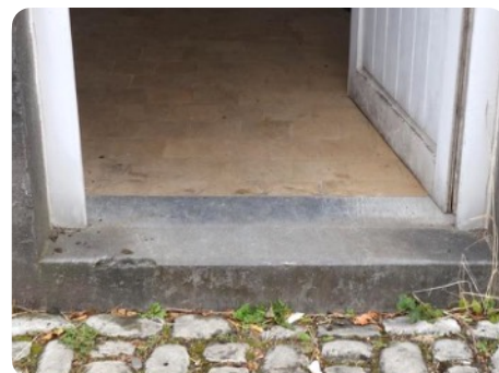
Blue stone door threshold (limestone)
