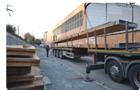
Transport of glulam beams
