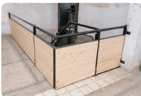
Conversion into guard railing, Brussels (BE) © Zinneke
