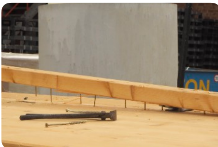
Removal of metal parts
