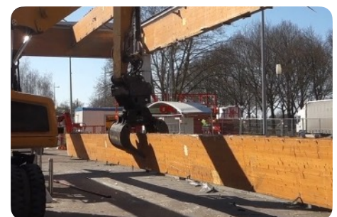
Removal of glulam beams
