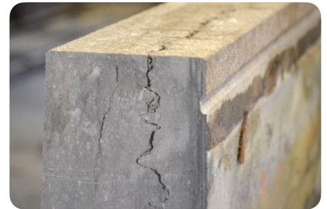
Example of stylolitic joints
