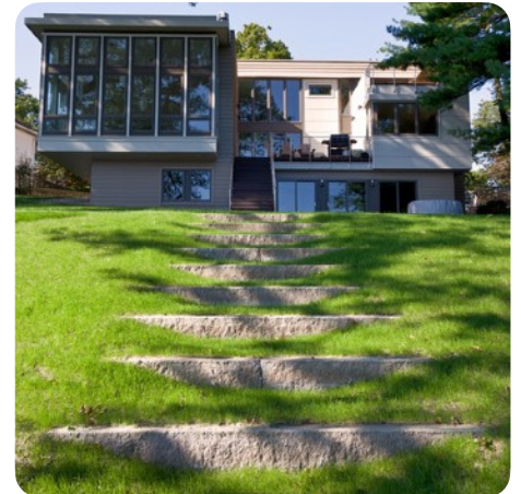
Lower Mystic Lake House (USA). Reclamation of stone kerbs. © matthew-cunningham.com
