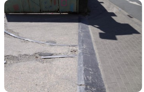
Lowered kerb profile
